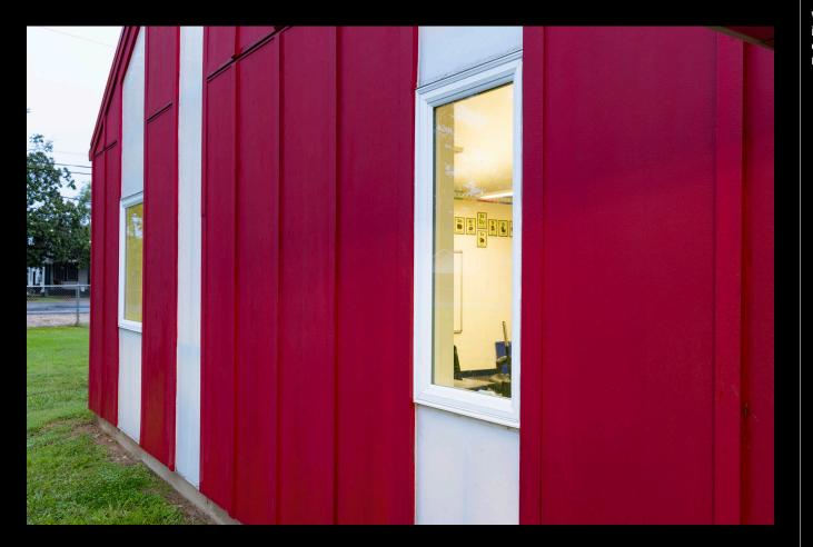
Z-flashing lines up with the top and bottom plates that show through the polycarbonate.
