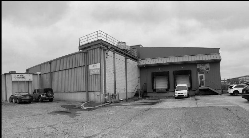
THE EXTERIOR CONDITION PRIOR TO RENOVATION
