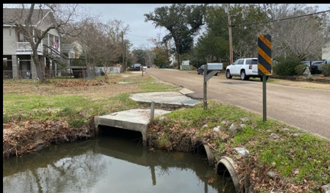
Ravine aux Coquilles channelized underneath Carroll Street
