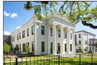
Finished renovations to the courthouse, flanked by new additions, in Spring 2023.
