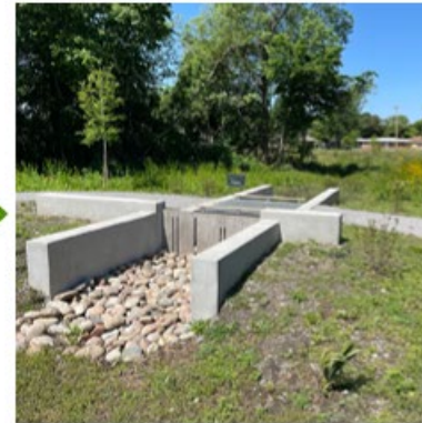
Water control structures interlace with the paths and landscape
